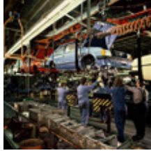
Final assembly (wedding) of an Opel Kadett D in the Bochum plant, 1979.
